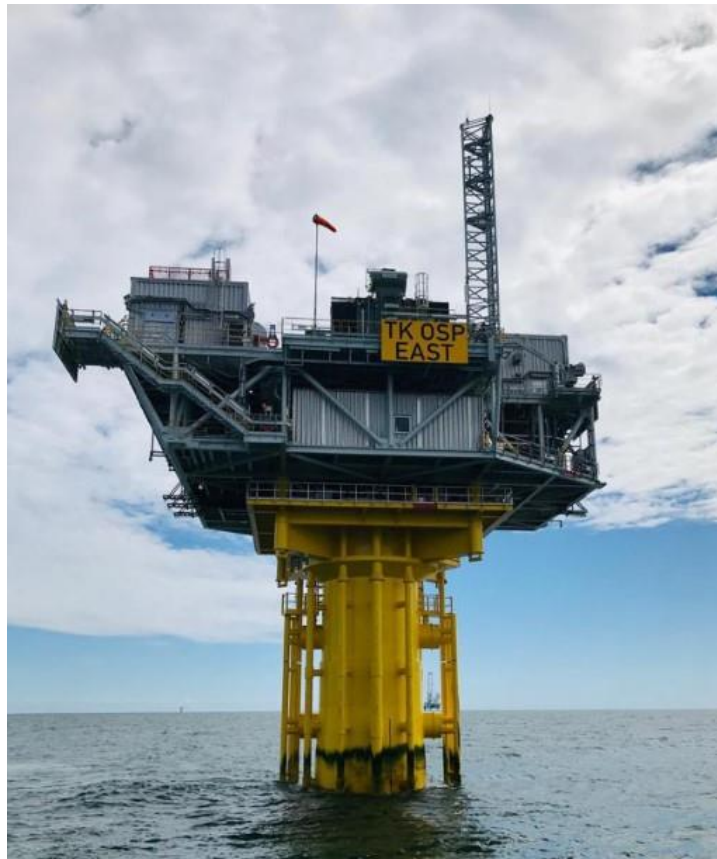
Plate 5-7 Example Offshore Platform from the Triton Knoll Offshore Wind Farm 6
